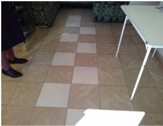
Picture 9; Inadequate repair in staff house
