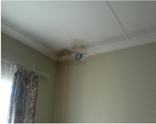
Picture 8; Leakage in staff house
