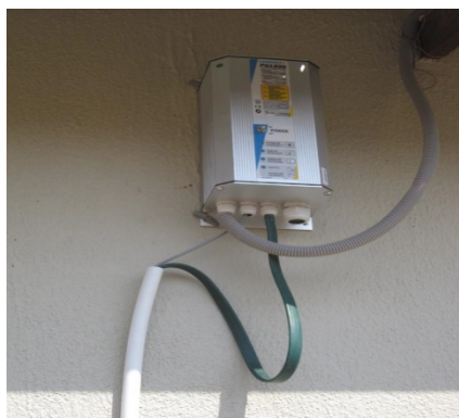
Picture 7; Inadequately fixed electric appliances.
